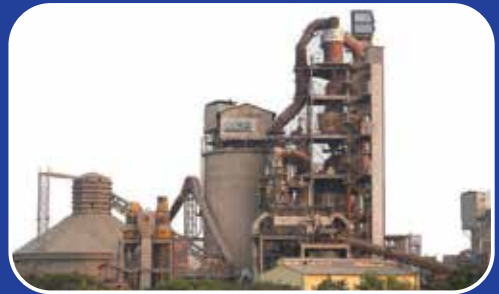
CEMENT PLANT MACHERLA
