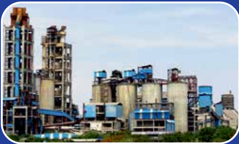
CEMENT PLANT MUKTYALA
